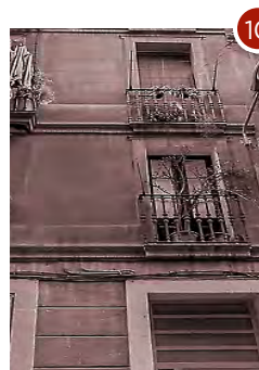
10 C. Pedreres Barcelona Sants-Montjuïc district
